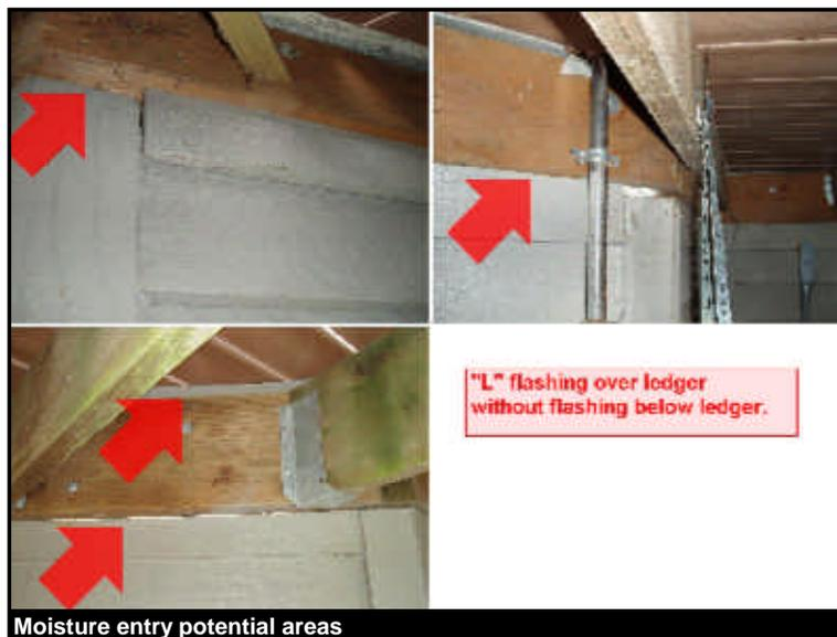
**Repair:** The "L" flashing present may allow water to get behind the ledger causing moisture damage as water can still get under the flashing. We recommend further corrective measures to keep water out.
