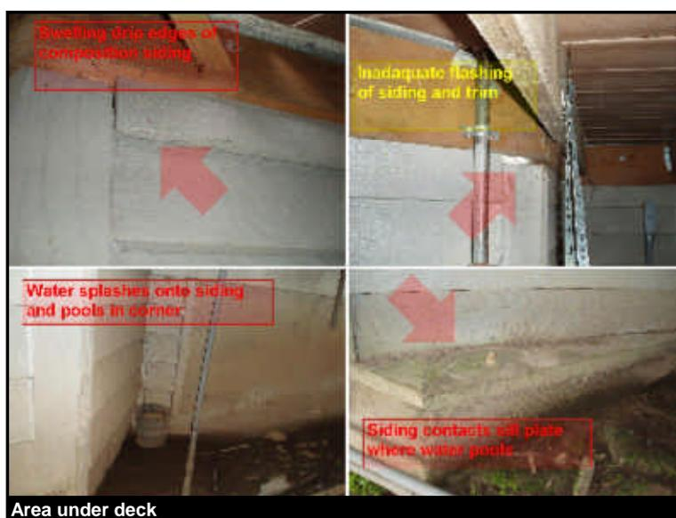
**Repair:** The drip edge of lap siding is separating and further siding damage is likely. We recommend that all deteriorated wood be repaired or replaced.
