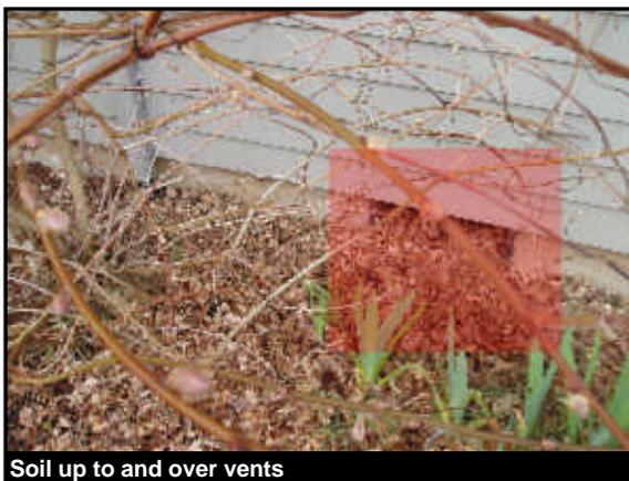
**Repair:** Crawlspace ventilation was observed to be below soil level. The bottom of the vent should be 4" above the soil level. We recommend clearing the vents for proper air flow of the crawl space and adding vent wells as needed to keep soil away.
