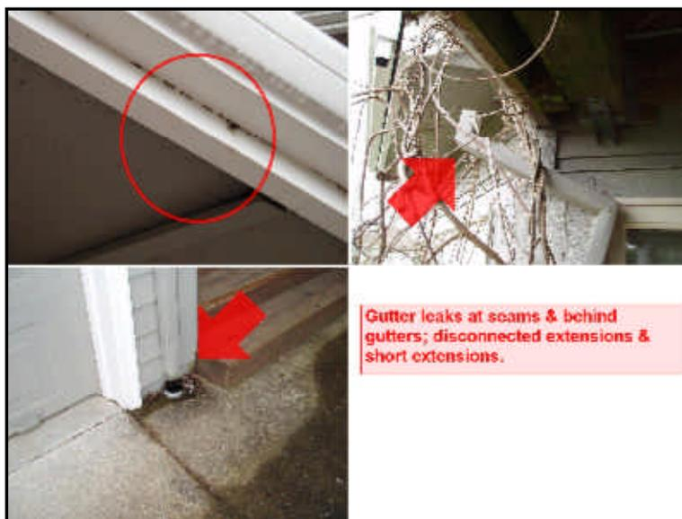
**Repair:** The gutters exhibit signs of leaks. We recommend that the gutters be repaired.
