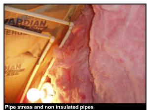
Repair: One or more water lines are not insulated in areas which are vulnerable to
