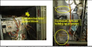
Maintenance: Dust and/or debris have built up on the blower and in the blower compartment. We recommend the blower and compartment be cleaned an the blower's bearing be lubricated.
