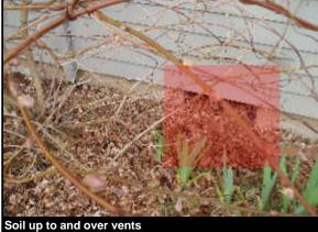
**Repair:** Crawlspace ventilation was observed to be below soil level. The bottom of the vent should be 4" above the soil level. We recommend clearing the vents for proper air flow of the crawl space and adding vent wells as needed to keep soil away.
